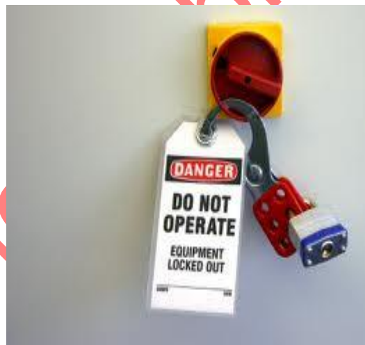
Figure 10 — An example of isolation: isolated switch
