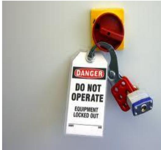
Figure 3 — An example of isolation: isolated switch
