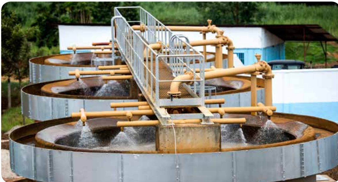
Nzove water treatment plant
