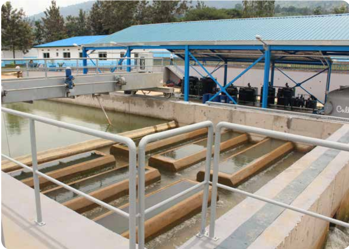
Nzove water treatment plant
